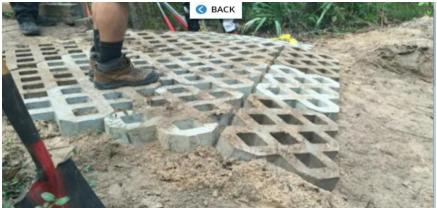
Volunteers not only repair the rail but mitigate the ongoing erosion from managing the water. Two Drain Dips were installed with Sedimentation traps.
