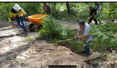
The Hiking element implemented Drain Dips in the Wilderness by hand. MUT volunteers applied the classroom training and dove into hands on reconstruction of drain dips in an attempt to stop erosion. Shoveling tons of soil has instilled a lasting appreciation for the impute of the drain dips.
